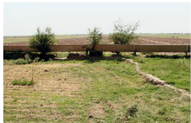
Fig. 3, 11 An elevated arık made of concrete, area of Gorintepa. Photo by Tereza Včelicová.
