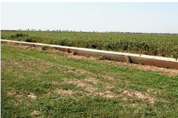
Fig. 3, 10 A concrete arık placed on the ground, area of Gilyambobtepa. Photo by Tereza Včelicová.
